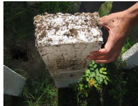
d) Investigated termite rating
