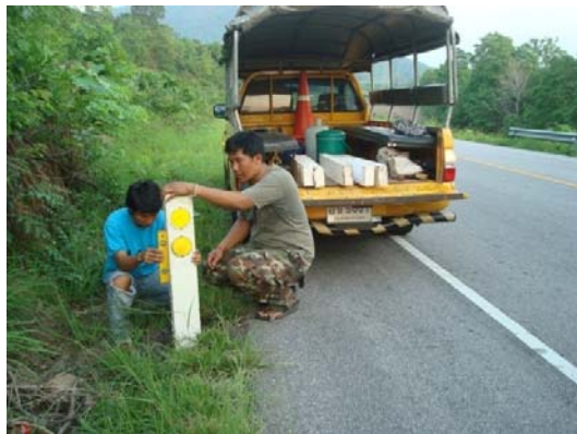
Figure 11 Application of eco-guide post on road number 104 in Wangchao-Tak region and road number 1090 in Maesord-Umphang region, Tak Province, Thailand.
