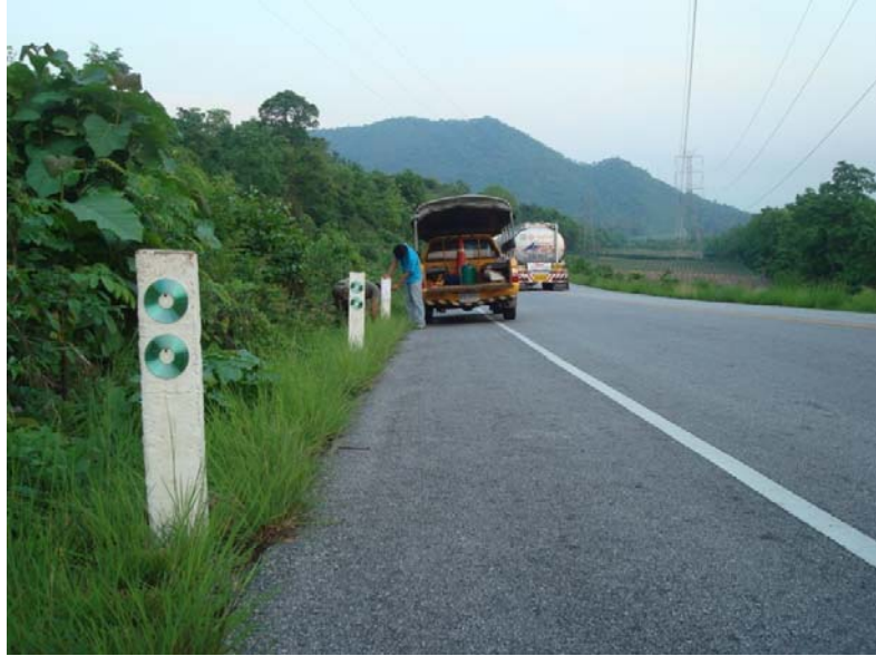
Figure 12 Eco-guide post version 1.1 improved by replacing reflectors with used CD
